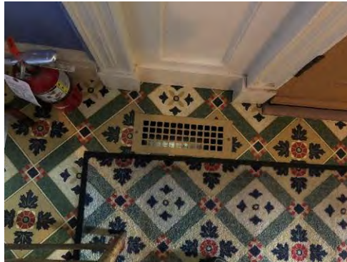
Typical First Floor Supply Register
