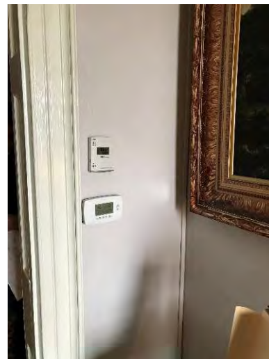
Typical Wall Mounted Thermostat and Wall Mounted Humidity Sensor
