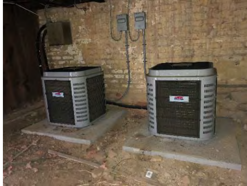
Air Cooled Condensing Units Serving AHU-1 and AHU-2
