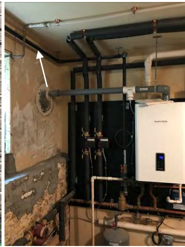
3/4" Gas Pipe Serving the Boiler
