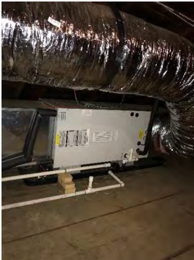
Horizontal Air Handling Unit AHU-2 Serving Second Floor
