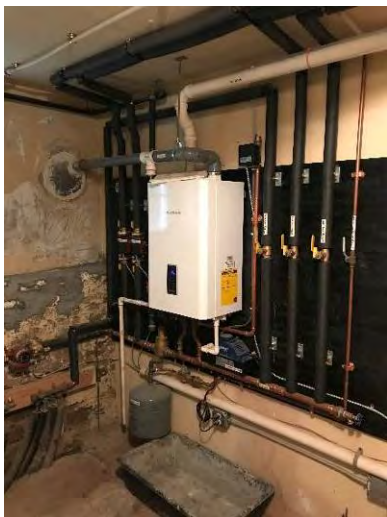
Wall Mounted Condensing Boiler B-1 and Associated Piping
