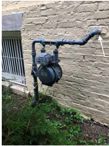
Gas Line Entering Basement
