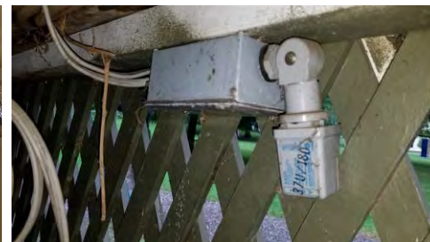
Exterior photocell for site lighting under south deck
