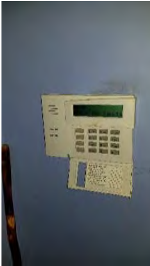
Security Alarm Keypad
