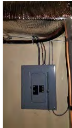
Mechanical Sub-panel
