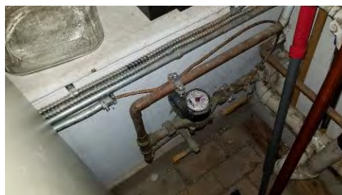
Electrical Grounding on Water Service in room B03.
