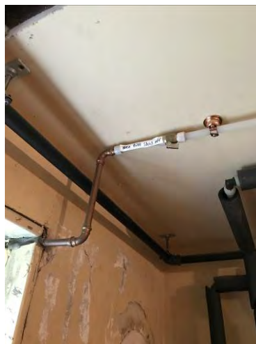
Copper and PEX Piping
