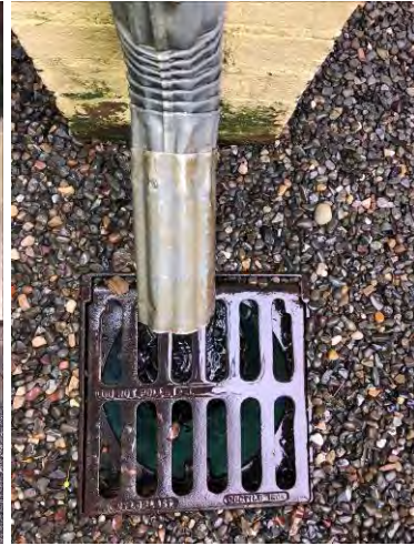
Open Grate to Storm Water System
