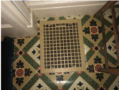
Main First Floor Corridor Return Register
