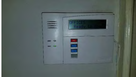
Fire Alarm key pad at main entrance
