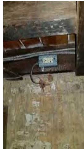
Exterior GFCI duplex receptacle
