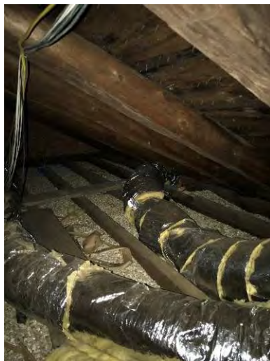
Flexible Ductwork in Attic Space
