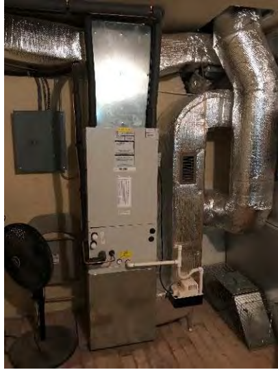
AHU-1 Serving the First Floor
