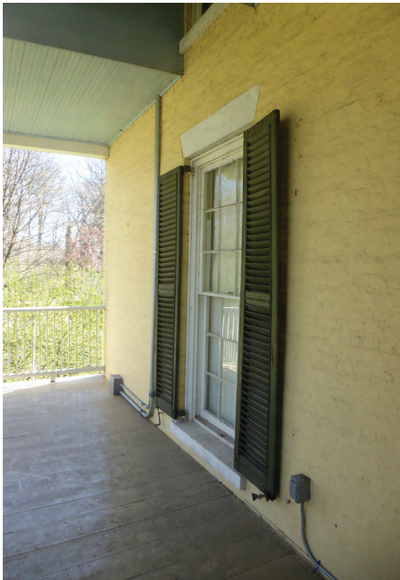
Figure 88. (Upper image) The low voltage wiring and cable routed along the façade of the north addition is visually obtrusive.
