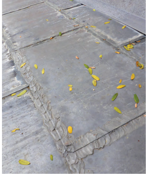
Figure 87. The excessive build-up of solder at the joints of the flat-lock seam metal roofing on the south porch has cracked. The soldered joints should be thoroughly sweated, so that solder flows freely into the seams. A cold joint, with solder build-up on the surface of the metal, does not provide serviceable performance. JGWA, 2019.
