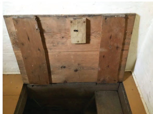
Figure 70. The cellar under 110, looking southeast (left) towards the window opening and the ladder-like stair. The image below shows the original floor hatch with its wood stock lock. JGWA, 2019.
