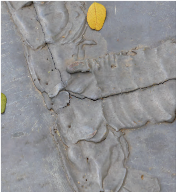
Figure 87. The excessive build-up of solder at the joints of the flat-lock seam metal roofing on the south porch has cracked. The soldered joints should be thoroughly sweated, so that solder flows freely into the seams. A cold joint, with solder build-up on the surface of the metal, does not provide serviceable performance. JGWA, 2019.
