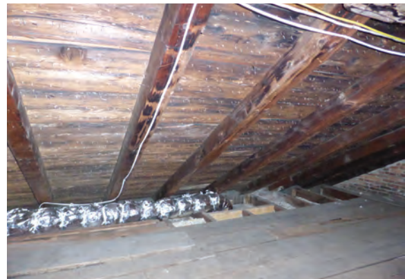
Figure 93. The paper and plaster ceiling and wall finishes in attic room 301 (upper image) are water-stained, dirty and cracked. Mildew appears to be growing on the walls in the northeast corner of the room. The roof rafters (lower image) are generally five inches wide and six inches deep, and spaced approximately thirty inches on-center. The roof structure may require reinforcement to adequately support snow loads. JGWA, 2019.
