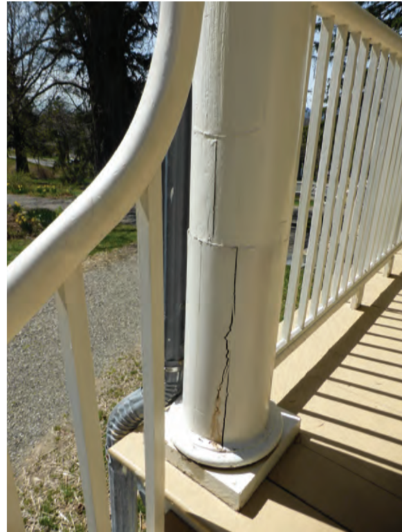
Figure 86. There are open seams in the repaired wood base of the southeast porch column. Water infiltration has caused rot and repair failure at several porch columns. JGWA, 2019.
