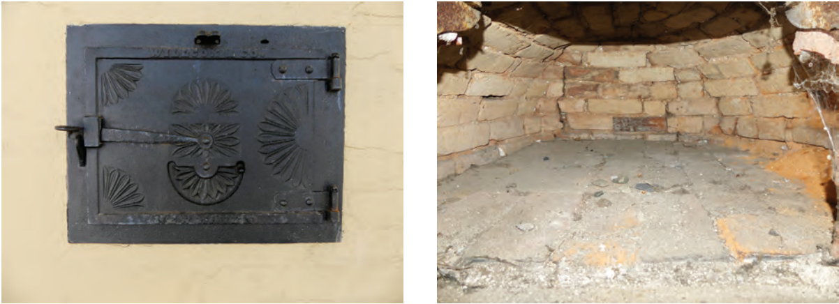
Figure 17. The bake oven door and chamber. The brick work at the far east end of the chamber appears to be the location of the original access from the 1815-16 kitchen. JGWA, 2018.
