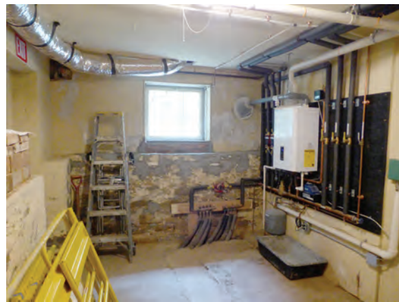
Figure 90. Heating pipes, manifolds and a gas-fired boiler have been surface-mounted to the walls at the southeast corner of Room B03. A fan-coil unit has been located at the west end of the room, and insulated ductwork has been routed throughout the space. The mechanical equipment thwarts historical interpretation of the space and increases the potential for fire. JGWA, 2019.
