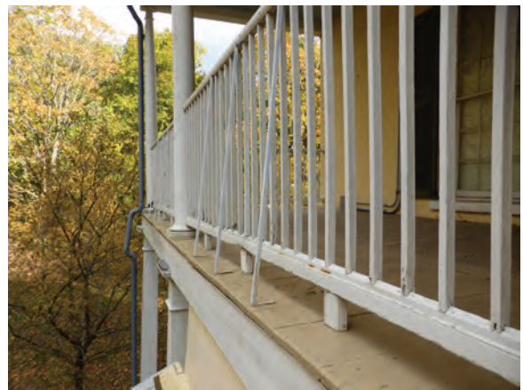
Figure 89. Northeast porch. Mildew is growing on the first-floor ceiling of the northeast porch (upper image). The wood railing is not well supported; it does not provide adequate resistance to lateral force, despite the addition of slender steel diagonal braces. The downspout at the northeast corner of the porch has broken loose of its attachment point on the post. JGWA, 2019.
